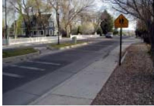
*Arterial road in Grand Junction, Colorado A median with a diagonal cut improves pedestrian access. Higher volume roadways require added crossing support. Note the added storage space, diagonal cut measures keeping pedestrians focused toward the traffic threat, and reductions in time of exposure.*
