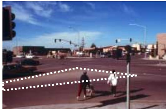
*Intersections designed for pedestrians should be compact, and produce low turning speeds. When care is not taken pedestrians are exposed to risks they cannot handle. Pennsylvania Avenue in Washington, D.C. is a model of excellenc. Meanwhile, this lower photo in Watsonville, California illustrates a missed opportunity. A channelized island location is indicated by debris markings.*
